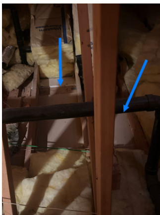
Image 8.1.1 Missing insulation
