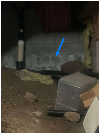
Image 7.2.1 Efflorescence
