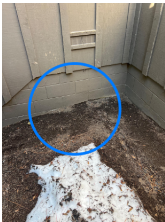
Image 1.5.1 Grading slopes towards foundation
